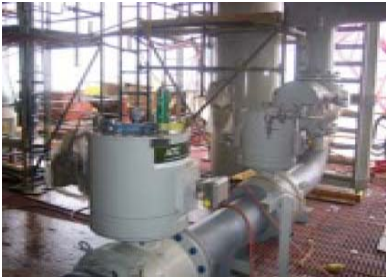
(Floating) Platform - 3 valves with ATC Spring Return Actuators, closely installed on horizontal and vertical mounted valves
